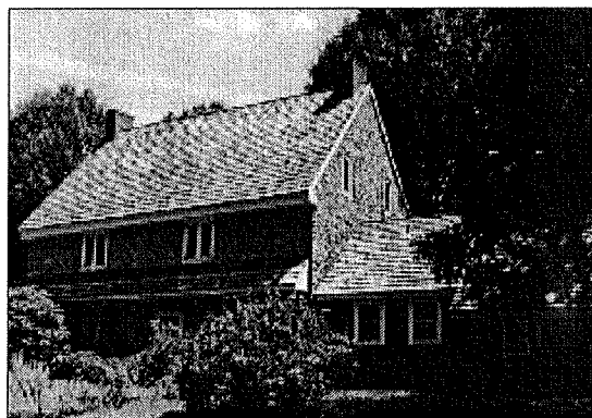
Isaac Watson House – Roebling Park, Hamilton Township Headquarters – Daughters of the American Revolution. Original construction - 1708
