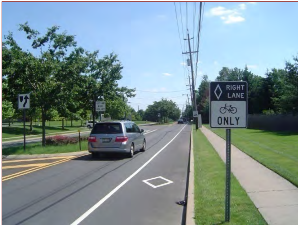
Federal City Road bicycle lane
