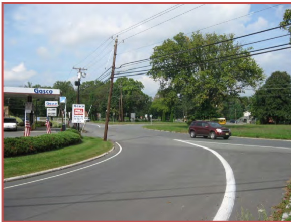
Exit lane from Route 31 Circle to CR 546 WB
