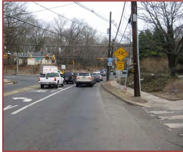
Wide shared through travel lane at intersection
