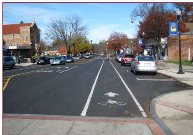
Example of a bicycle lane facility in a town center
