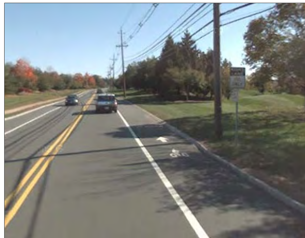
Bicycle lanes striping on a county road in Somerset County
