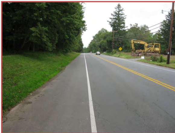
8’ wide paved shoulder on CR 546
