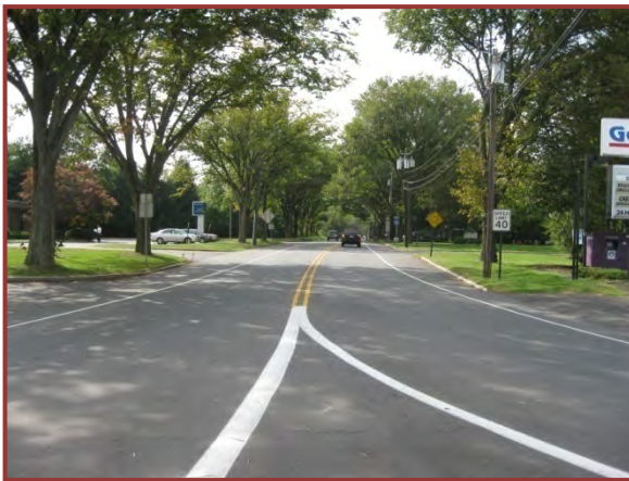
Route 546 to the west of Route 31 Circle
