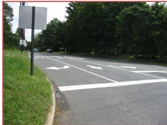
Lane configuration on the east side of the intersection of CR 546 and CR 579
