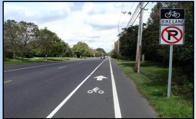
Above: Standard bike lane in West Windsor, NJ Source: Jerry Foster
