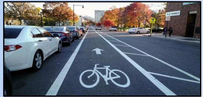
Above: Buffered bike lane on Warren Street in the City of Trenton, NJ. Source: Jerry Foster
