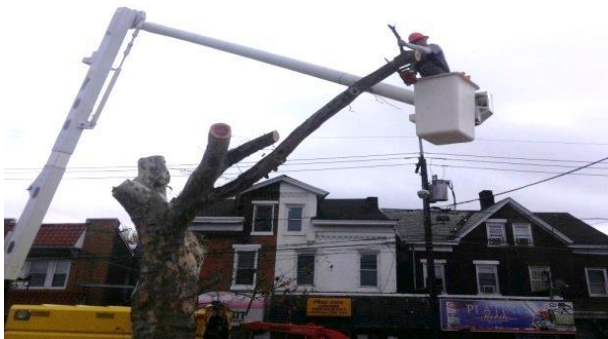
Removal of a large Sycamore Tree on Hamilton Avenue @Chambers Street in the City of Trenton to provide clearance for the new McDonald's.
