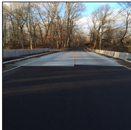
Above: Bridge No. 672.9, Tattletown Road, completed.
