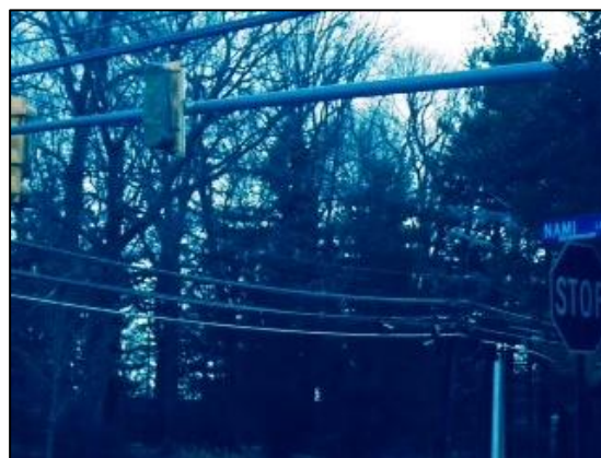
Above: New traffic signal at Quakerbridge Road and Nami Lane.
