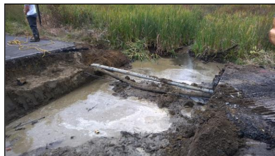
Above: South Post Road Culvert (742.1) excavation
