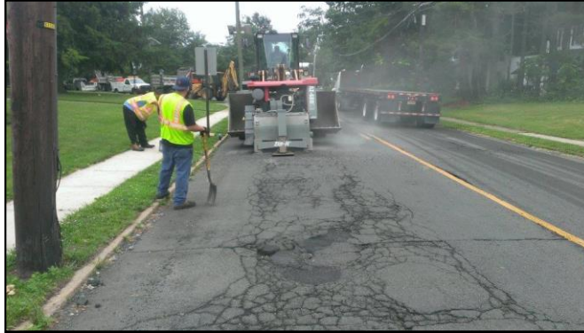
Above: Pothole Repair on Grand Ave. in Ewing Township
