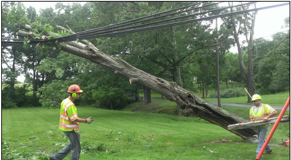
Above: Tree obstructing wires on Pennington-Harbourton Road.
