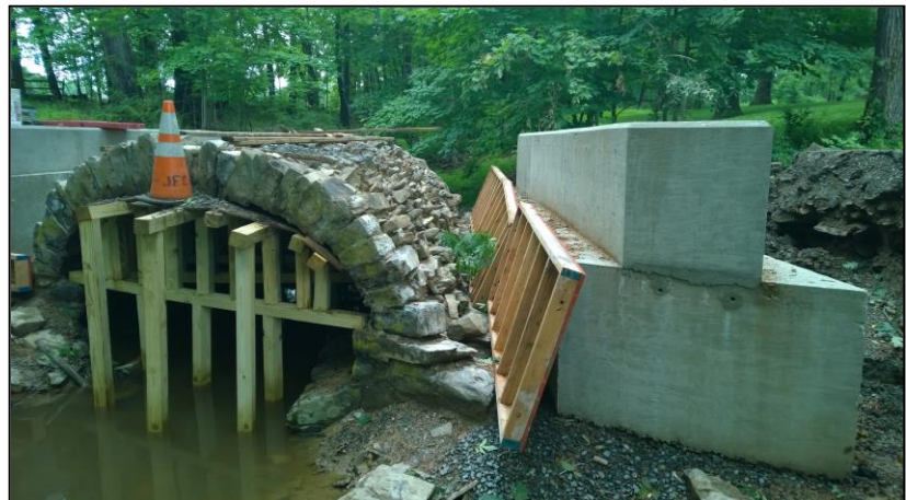
Right: Existing stone arch supported during Van Dyke Bridge (234.1) reconstruction.
