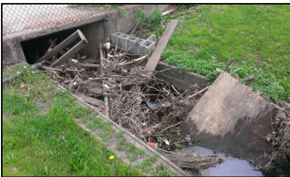
Left: Debris clogging raceway. Service request received from residents.
