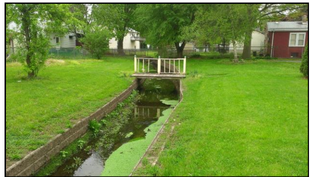
Left: Debris clogging raceway. Service request received from residents.
