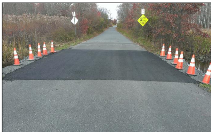
South Post Road Culvert (742.1) replacement complete
