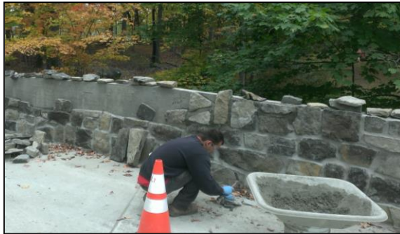
Left: Van Dyke Bridge (234.1) parapet wall reconstruction.
