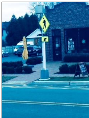
Left: Rectangular Rapid Flashing Beacons Installed at East Broad Street at the Farm Market, Hopewell Township.
