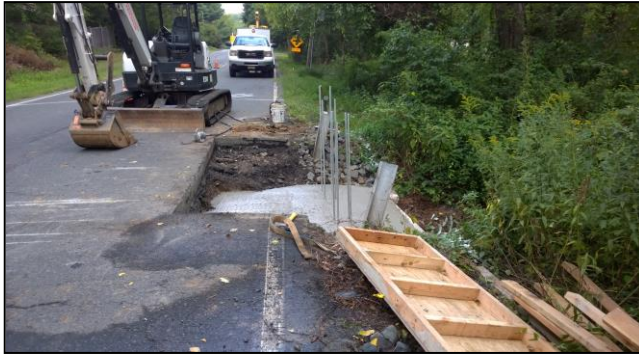
Left and Below: Lambertville-Hopewell Rd Culvert (234.12) emergency repair in progress.
