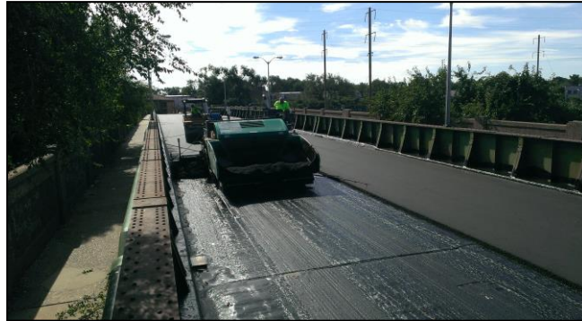
Above: Rehabilitation of Lincoln Avenue Bridge in the City of Trenton
