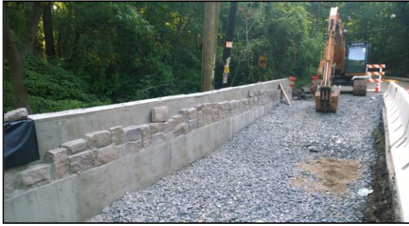
Above and Right: Bear Tavern Road Bridge over Jacobs Creek (214.2) wall reconstruction.
