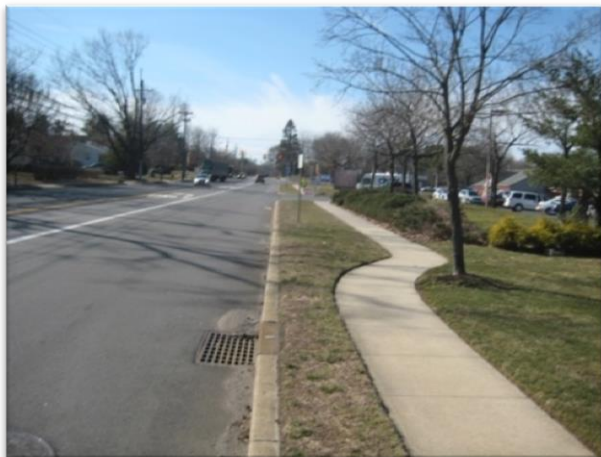
Above: Intersection Improvements @ Quakerbridge and Youngs Roads, Hamilton Township
