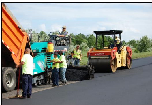
Below and Right: Milling and Resurfacing Scotch Rd. (CR 611) in Hopewell Township
