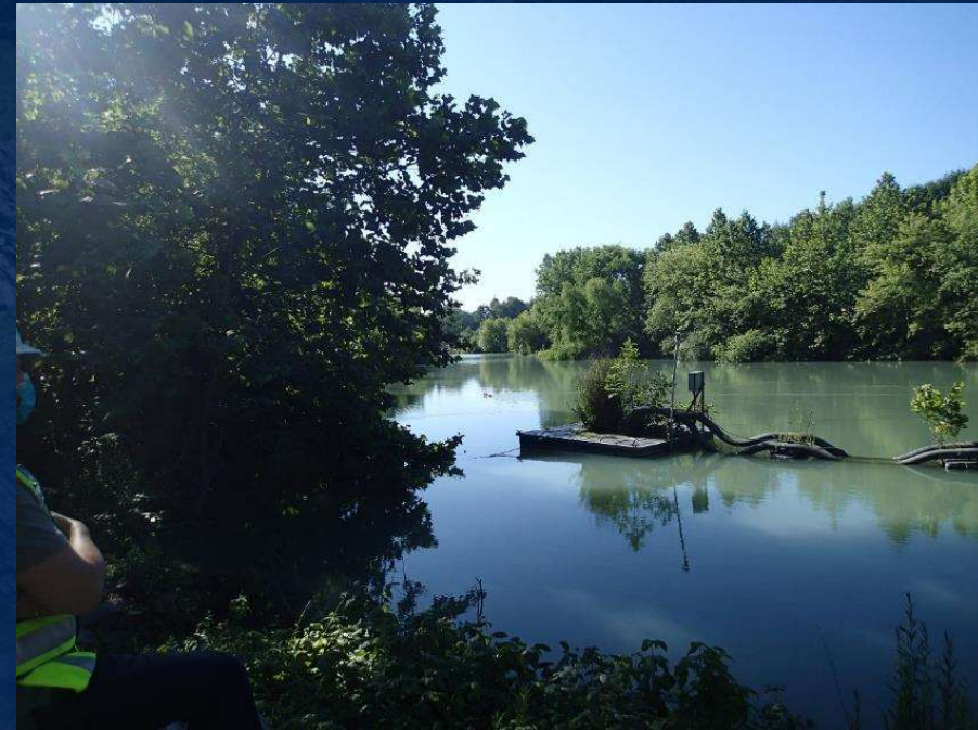
Site pond used for dewatering pit and dust control
