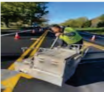
Pictured above: Yellow thermoplastic gore markings are angled for roadway delineation application
