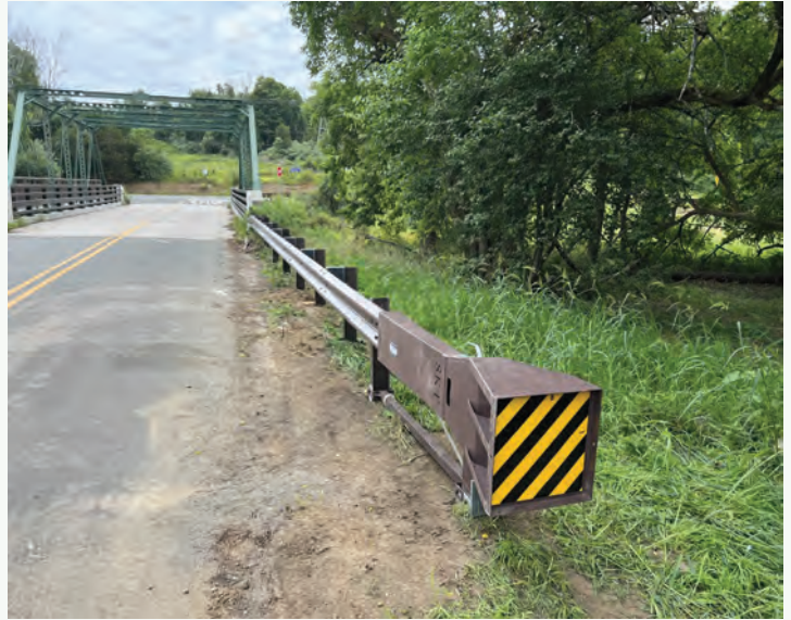
Pictured above: Valley Road in Hopewell Township after full replacement
