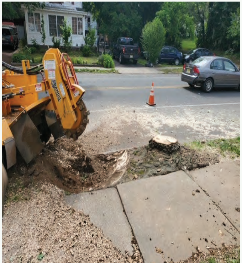
Pictured above: Stump grinding at 837 Parkside Avenue in Ewing Township
