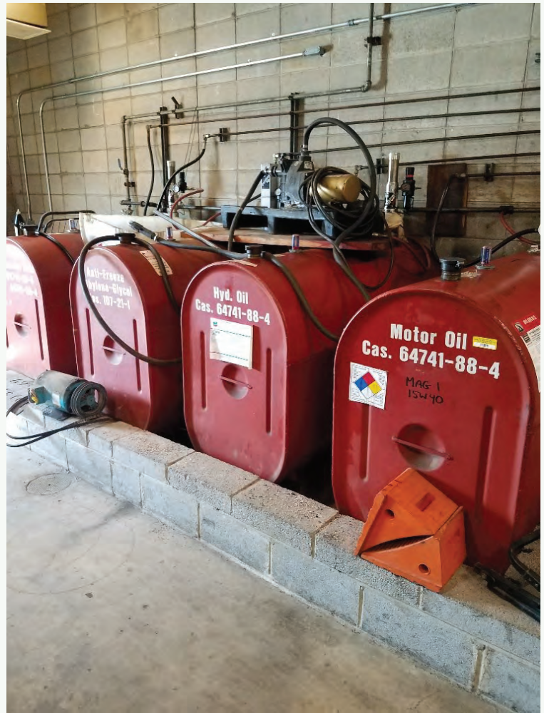
Pictured above: Replacement of Lubrication Pumps
