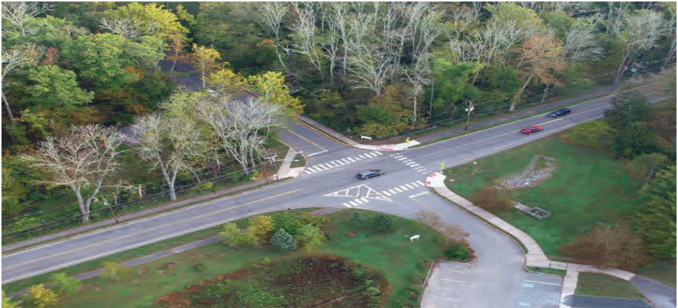
Pictured above: Previous condition at Rosedale Road and General Johnson Intersection in Princeton
