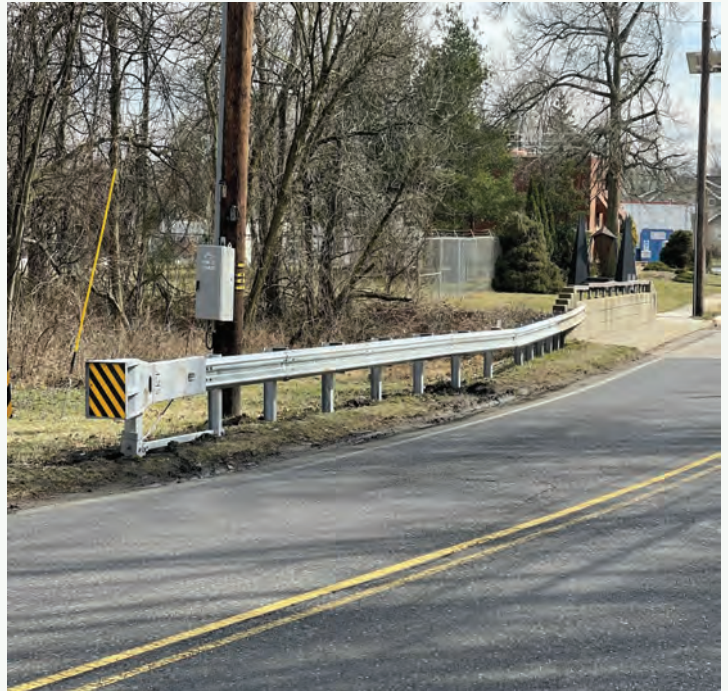
Pictured above: Klockner Road in Hamilton Township after repairs in March 2022
