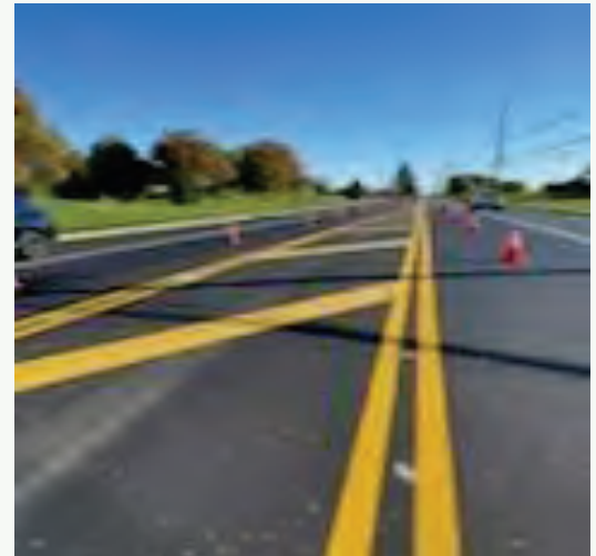
Pictured above: Yellow thermoplastic gore markings are angled for roadway delineation application
