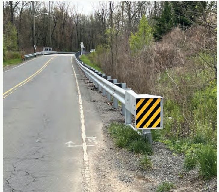
Pictured above: Basin Road in Lawrence Township after repair in April 2022
