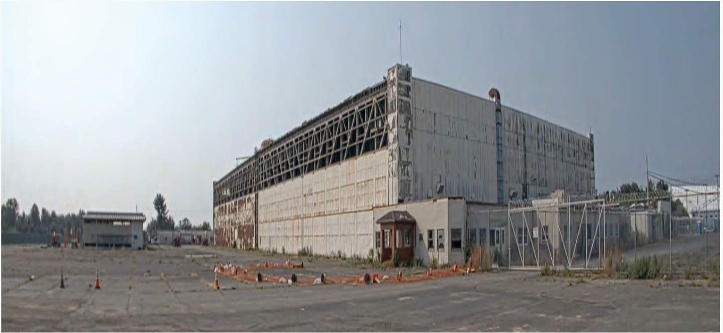
Pictured above: Old Navy hangar prior to demolition
