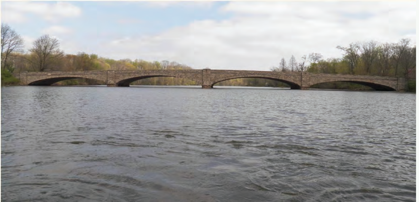
Pictured above: Washington Road Bridge (Structure No. 360.1), Princeton
