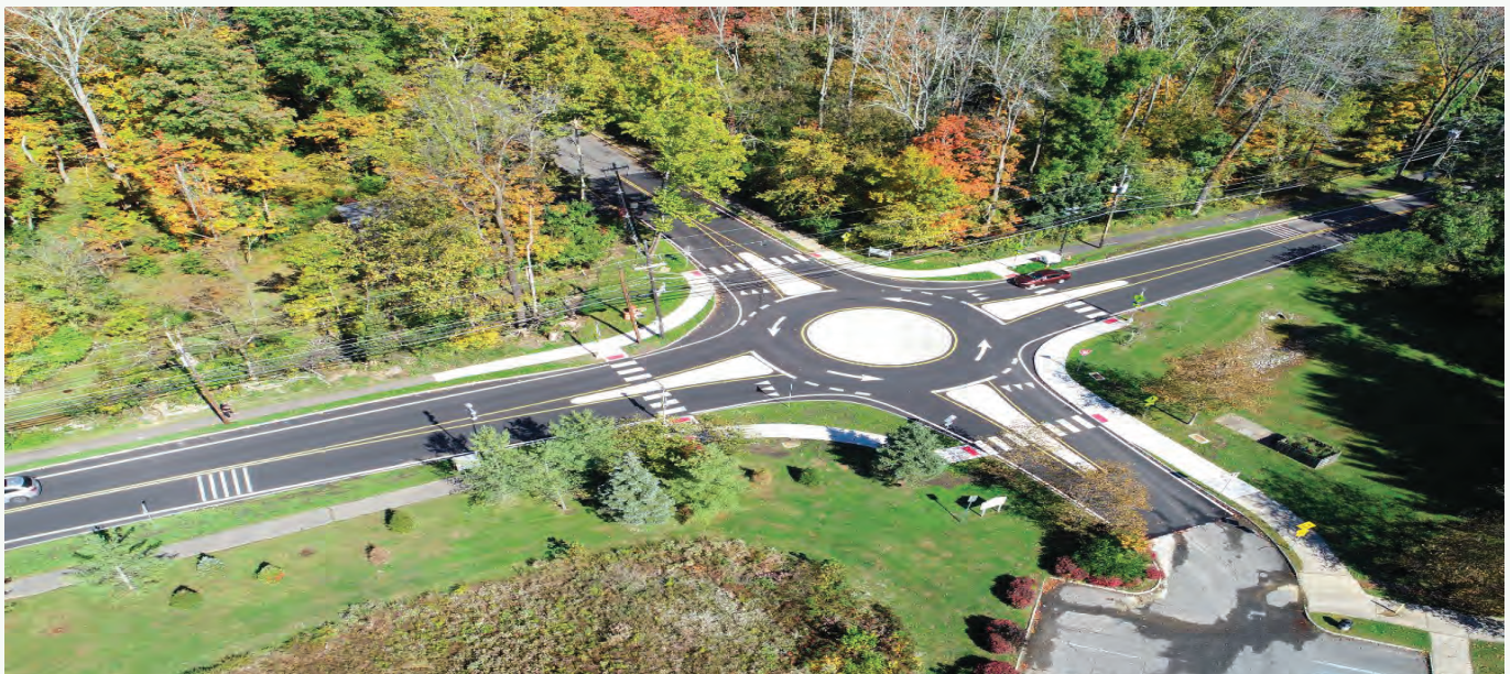
Pictured above: Newly installed Mini-Roundabout at Rosedale Road and General Johnson Intersection in Princeton
