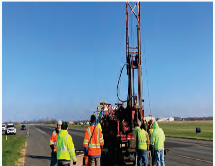
Pictured above: Core samples being taken on Taxiway A
