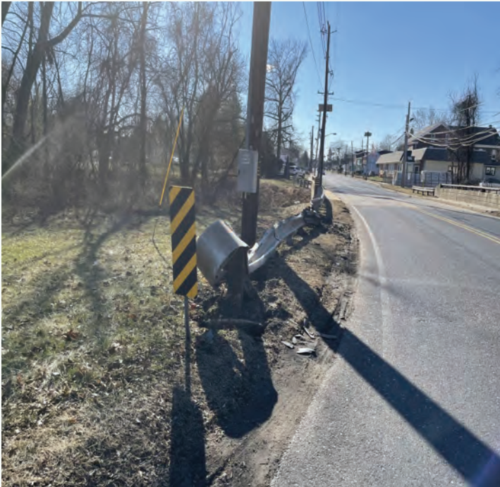
Pictured above: Klockner Road in Hamilton Township, guiderail was hit on its tangent terminal
