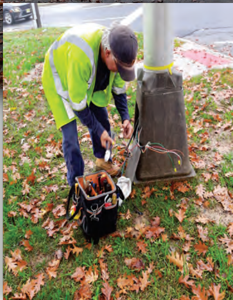
Pictured right: Senior Traffic Signal Electrician, Richard Danley makes wire connections
