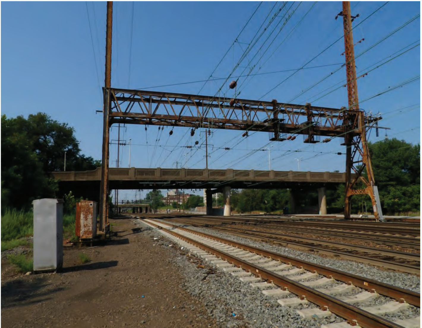
Pictured above: Lincoln Avenue Bridge (Structure No. 140.9), City of Trenton
