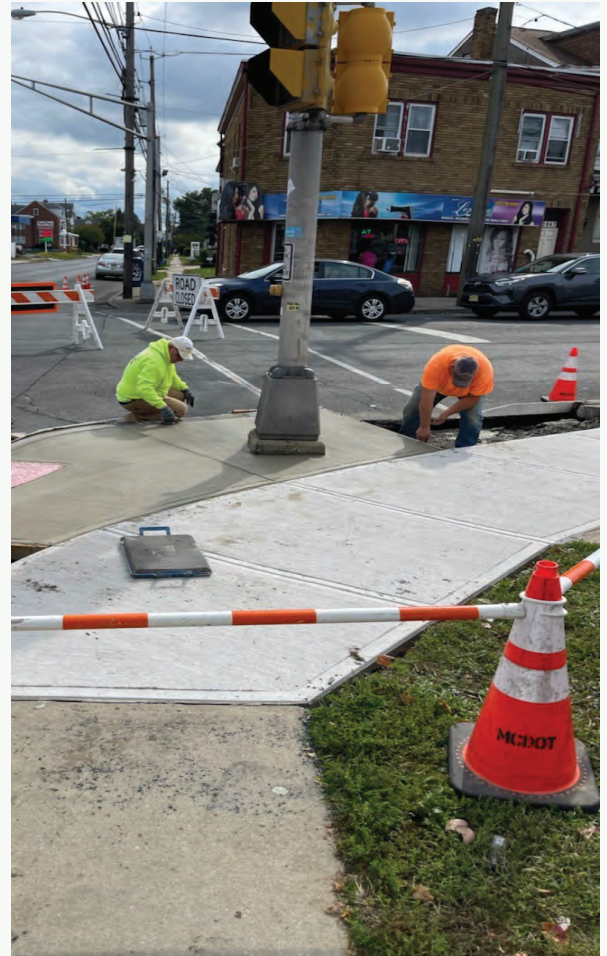
Pictured above: Chambers Street, Hamilton Township
