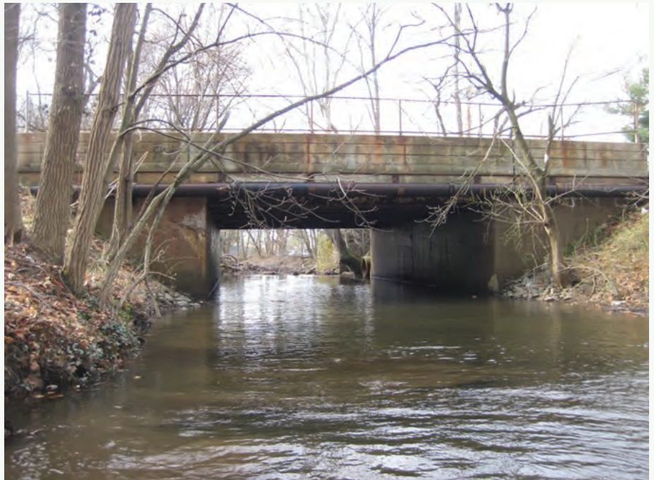
Pictured above: Elevation view (Structure No. 641.4) , Hamilton Township
