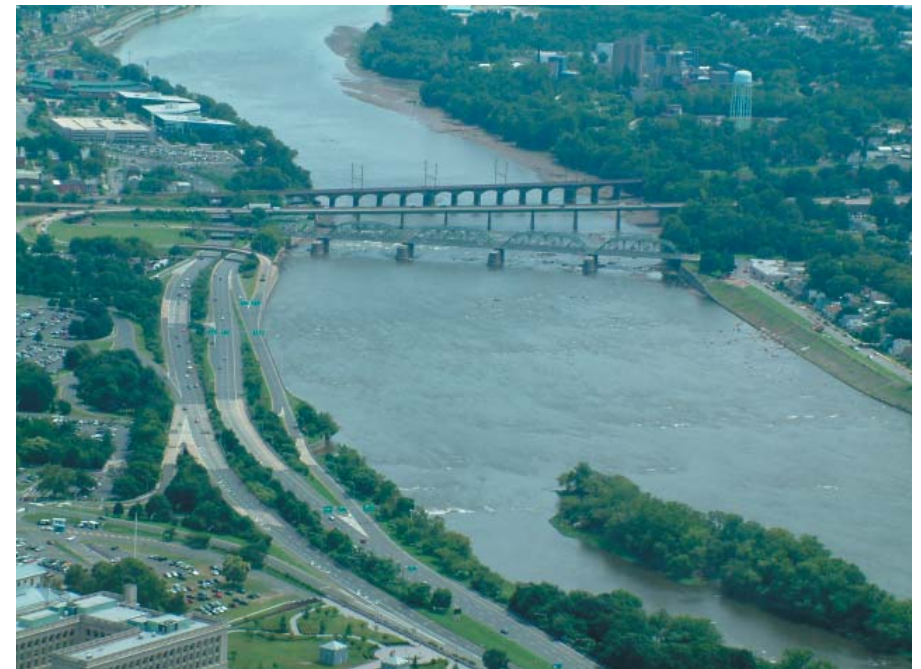
Highway access ramps are being reconfigured to US1 by the Delaware River Joint Toll Bridge Commission to make them more compatible with the more urban street network and to free up land in the downtown.
