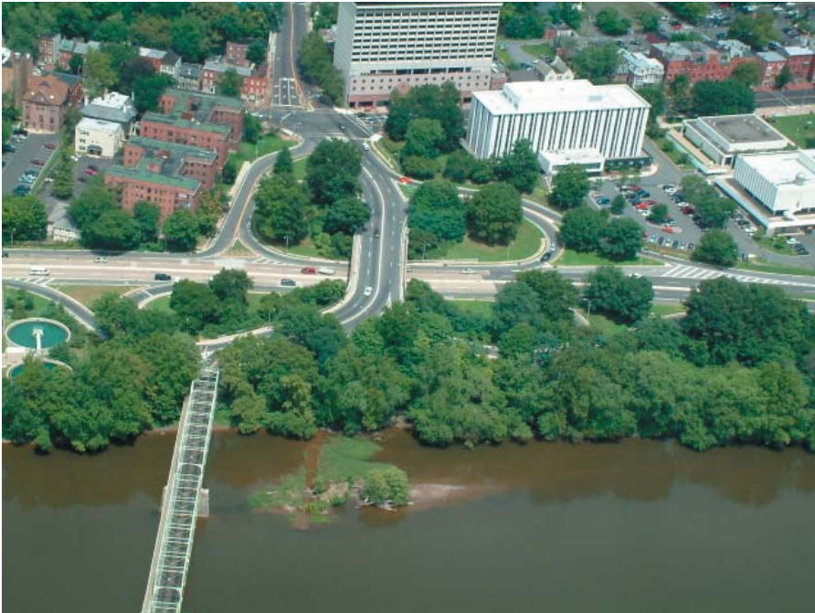
The Calhoun Street bridge ramps promote speed, poor aesthetics, and consume a considerable amount of real estate.
