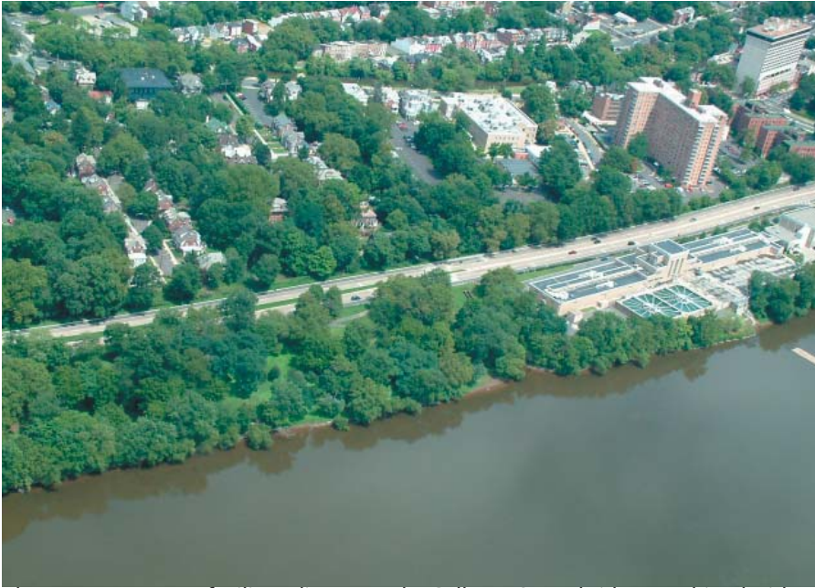
The water treatment facility, adjacent to the Calhoun Street bridge, combined with the long, straight, and flat section of Route 29 are formidable obstacles to getting to the river.
