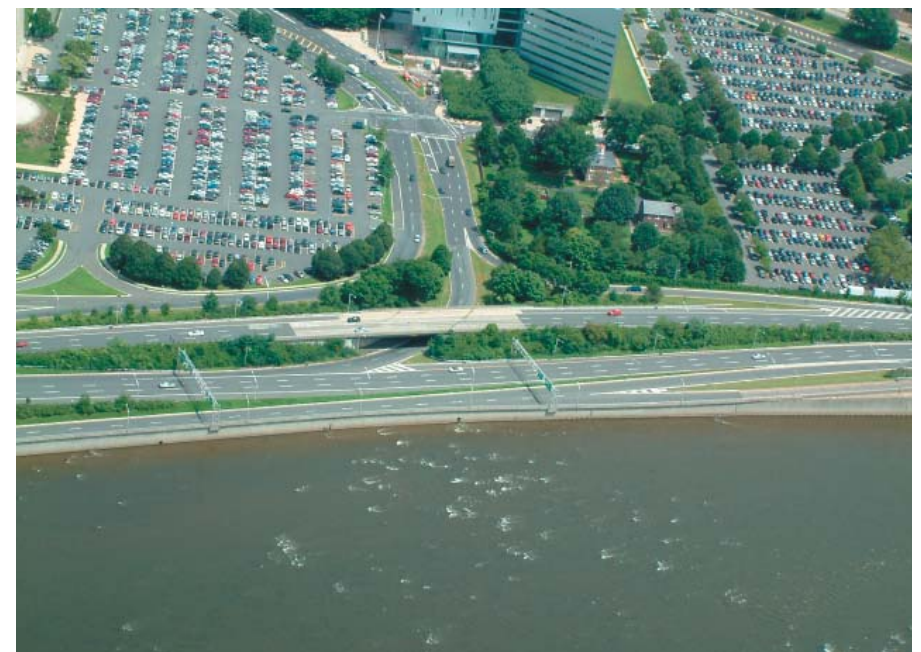
Market Street serves as a highway access ramp to Route 29 and a circulation route for the adjacent surface parking lots.
