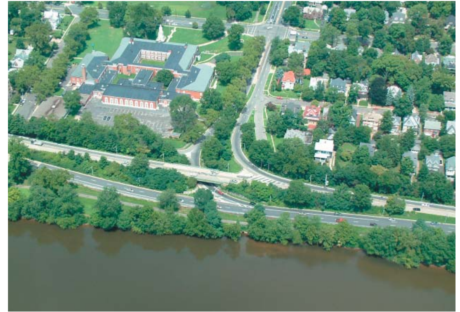
The high speed ramps connecting northbound Route 29 to Parkside Avenue.
