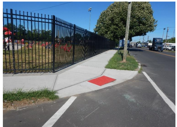
New Sidewalk and Curb Ramp by Capital City Sports Complex
