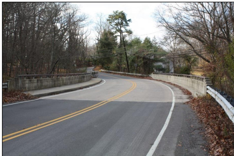
Existing Cranbury Road (Bridge No. 762.1)
