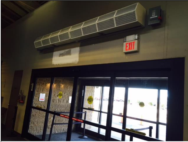
Trenton – Mercer Airport New air curtain installation
