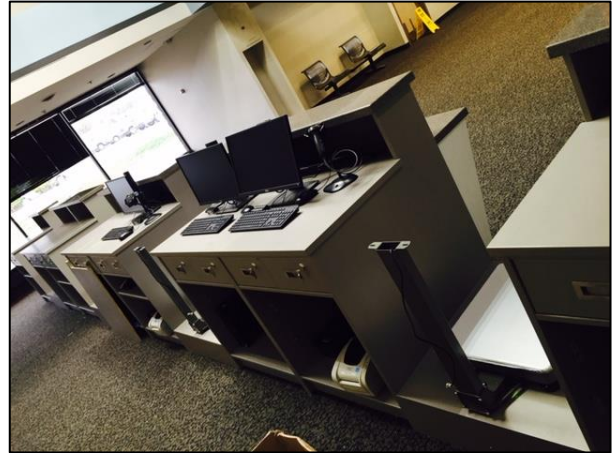
Trenton – Mercer Airport New ticket counter installation
