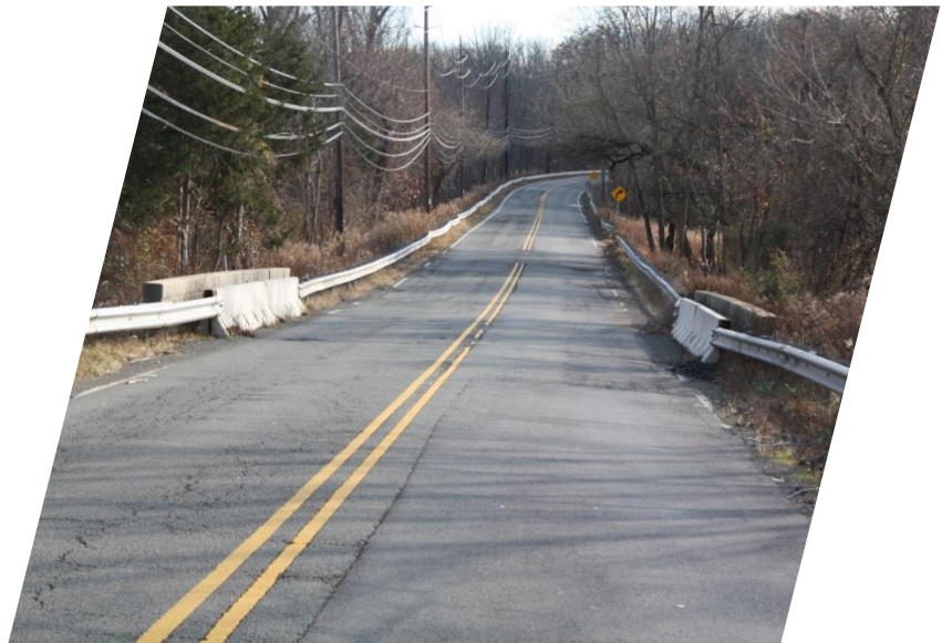
Existing Carter Road Bridge (No. 250.3)
