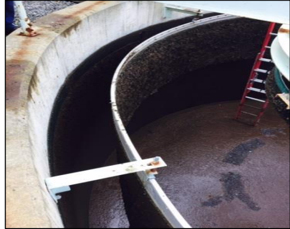
Sewage Treatment Plant Clarifier Repair
