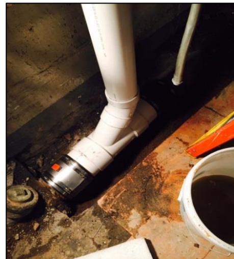
McDade Administration Building Main sewer line repair
