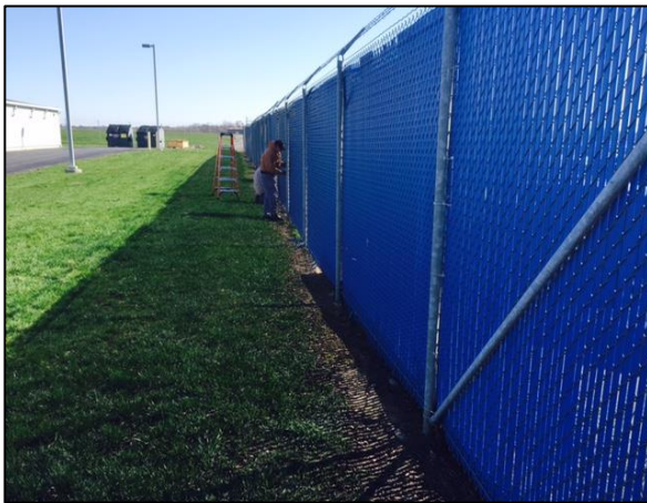
Prosecutor's Office Fence Repairs
