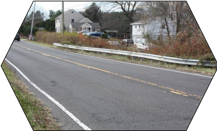
Existing Old Trenton Road (Bridge No. 745.3)
