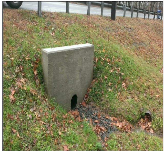
Pennington-Hopewell Road (Bridge No. 235.1) Installation of new headwall
