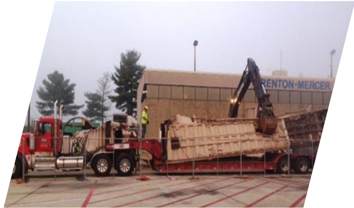
Retired jet bridge being loaded for removal
