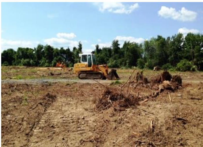
Removal of trees that were negatively impacting aircraft navigation
