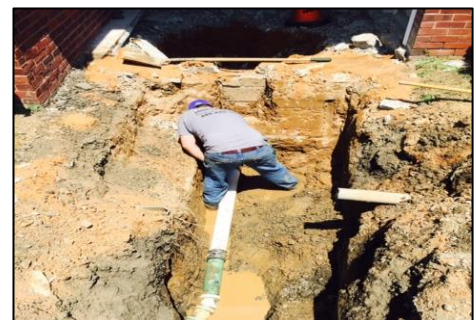
Veteran's Building Sewer line repair
