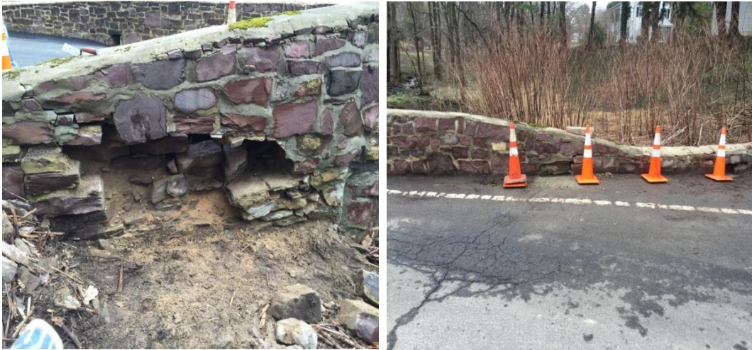
Quaker Road (Bridge No. 332.2) Completed parapet wall
