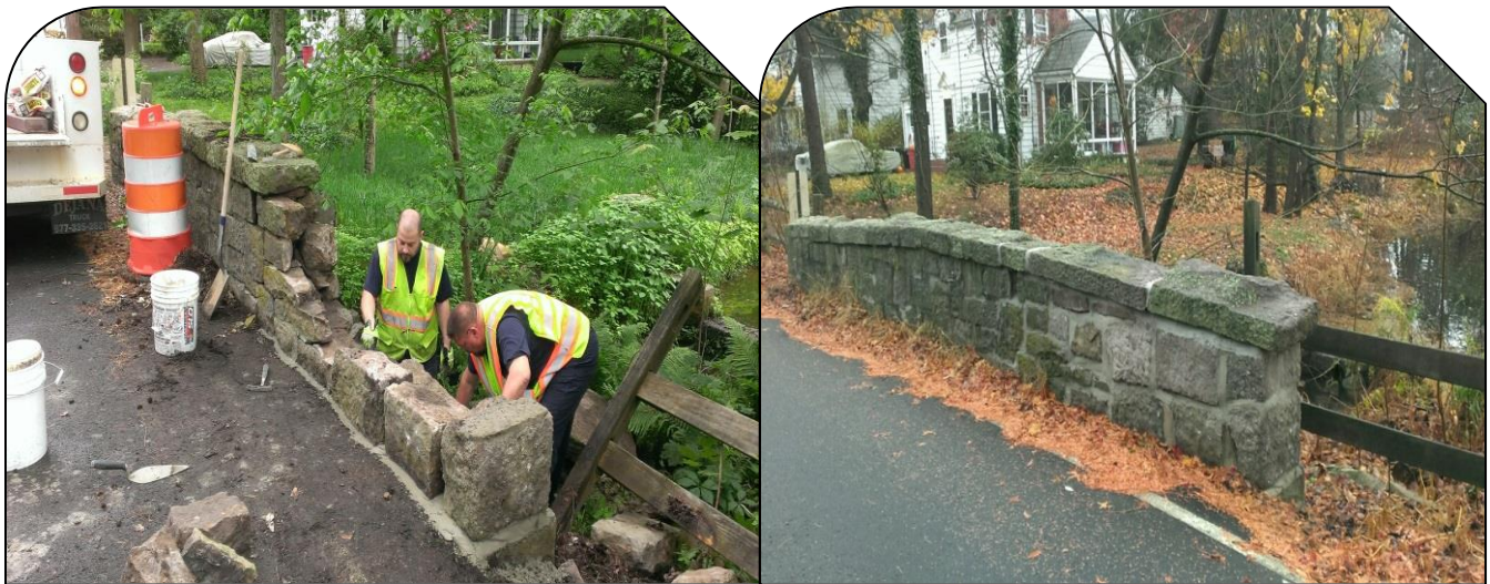
Structure 411.1 – Wilburtha Road Bridge Unit personnel repairing stone parapet wall
