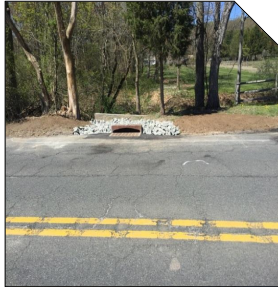
Structure 212.9 – Bear Tavern Road Completion of new inlet and pipe
