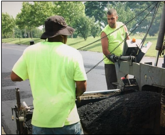
Resurfacing Project Road Unit Personnel
