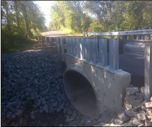
Dublin Road (Bridge No. 216.17) Completed the removal/replacement of elliptical pipe
