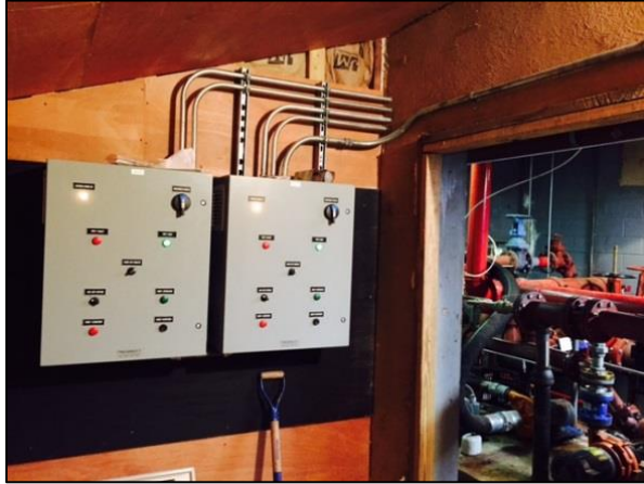
Correction Center Upper Pump House Variable frequency controls replacement
