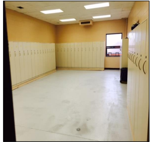
DOT & I Facility Locker room renovation
