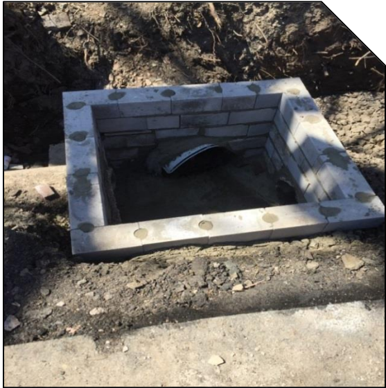
Structure 212.9 – Bear Tavern Road Completion of new inlet and pipe
