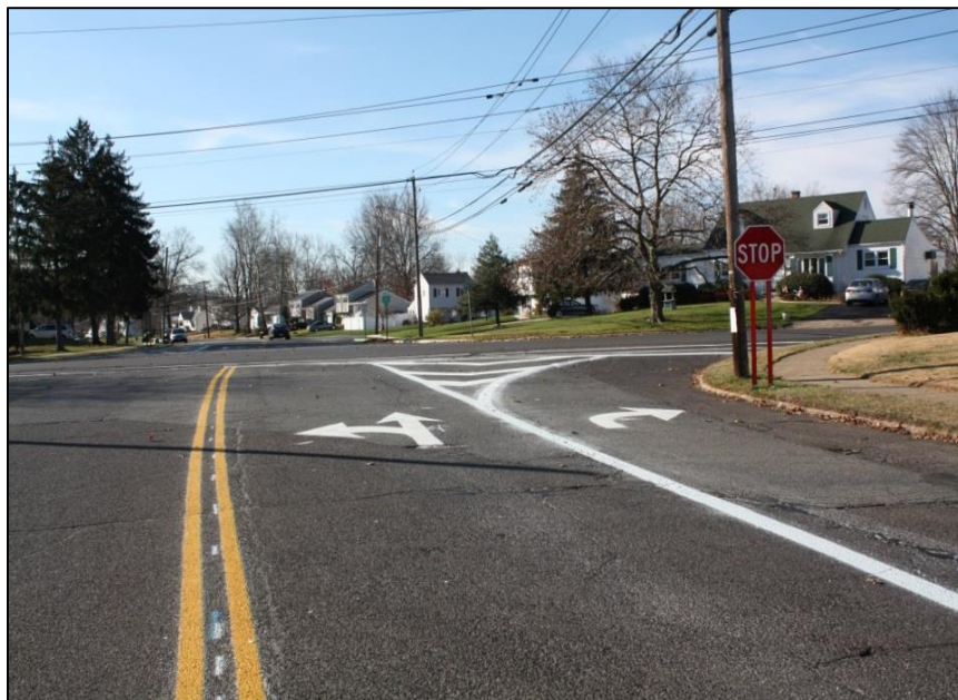
New pavement markings on Hempstead Avenue at Arena Drive
