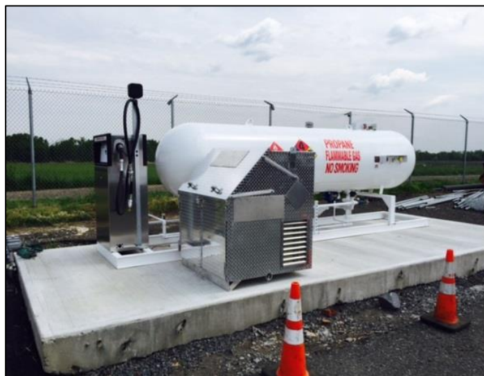
Motor Pool New propane station installation
