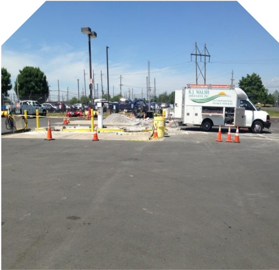
Contractor R.J. Walsh Associates Replacement of tank sumps and piping
