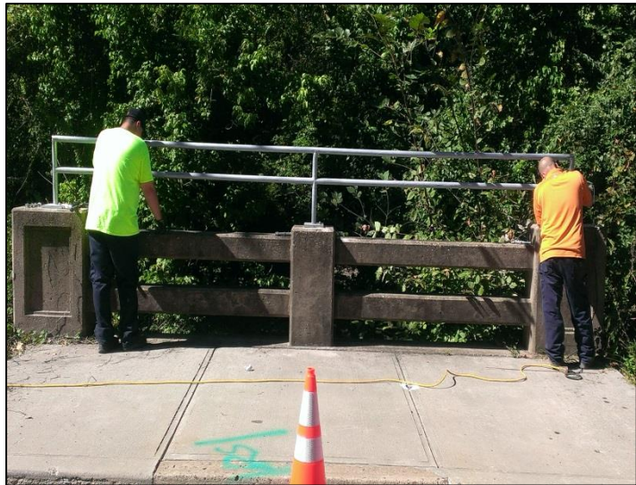
Great Road (Bridge No. 335.8) Bridge Unit personnel installing new parapet rails
