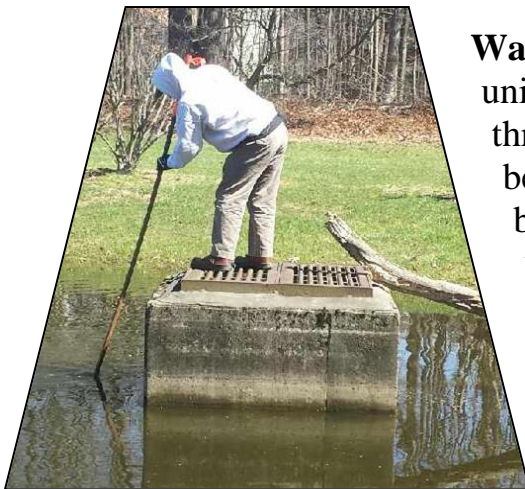
Above: Water Management unclogging a detention basin allowing water to flow.
