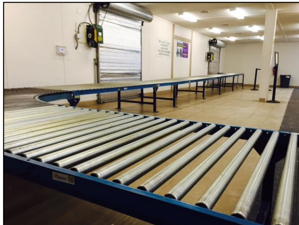
Trenton – Mercer Airport New baggage claim system installation
