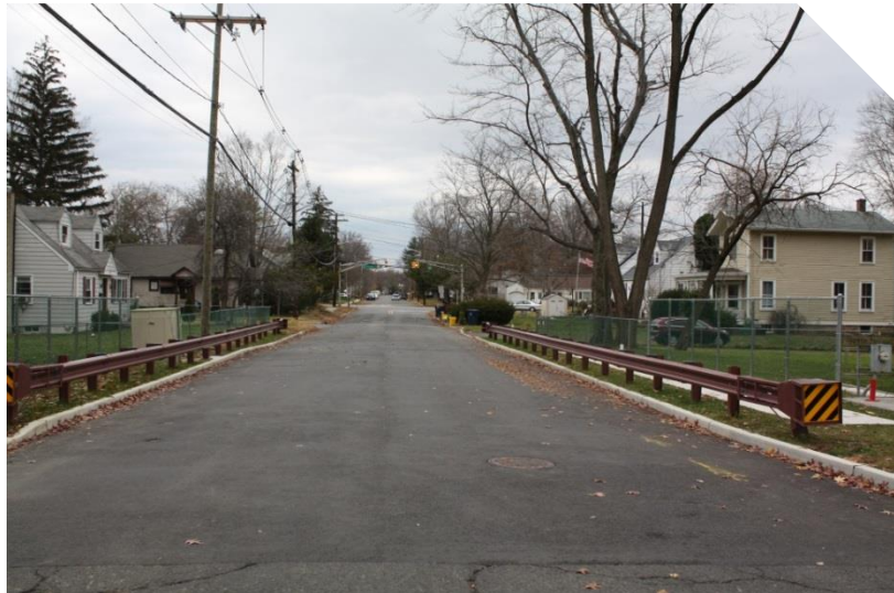
Maxwell Avenue (Bridge No. 863.10) Completed construction
