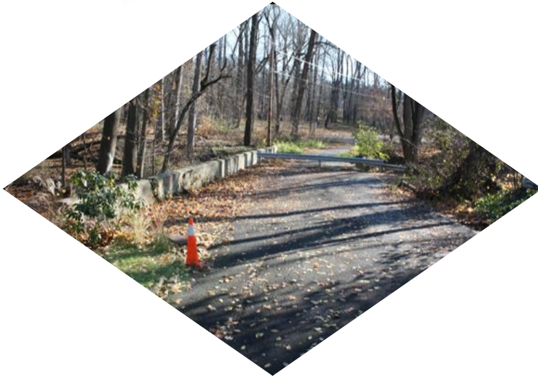
Existing River Drive Bridge closed to traffic for start of construction
