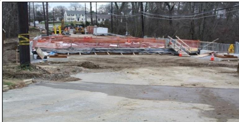
South Broad Street Bridge (No. 672.4) During construction
