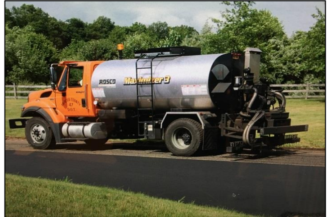
Maximizer 3 Applying liquid asphalt
