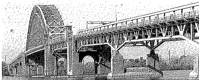
Built in 1928–29, the Tacony-Palmyra bridge over the Delaware River was one of many spans for which the American Bridge Company supplied structural steel. [Hunter Research, Inc.]
